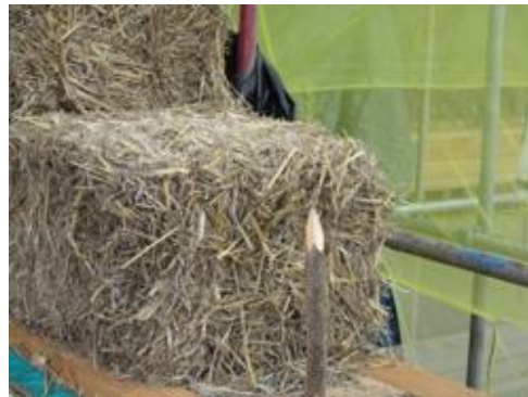
Picture 3: Hazel 'stub' stake in the base plate ready
