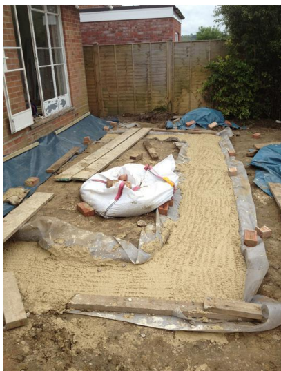
Fig 21 Ready-mix limecrete foundation for a new conservatory Photo: the.woodlouse.blogspot.com
