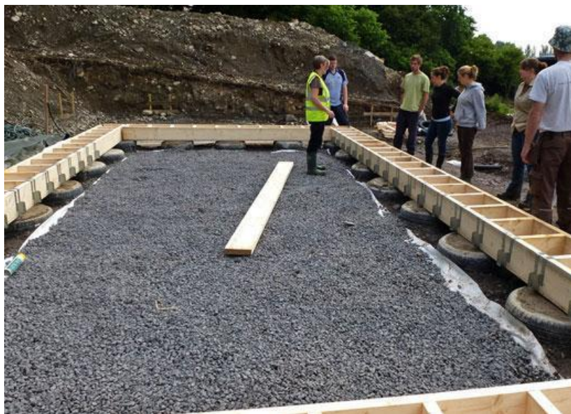
Fig 24 Box beam on rammed tyre foundations, Suffolk straw bale cottage Photo Strawbuild
