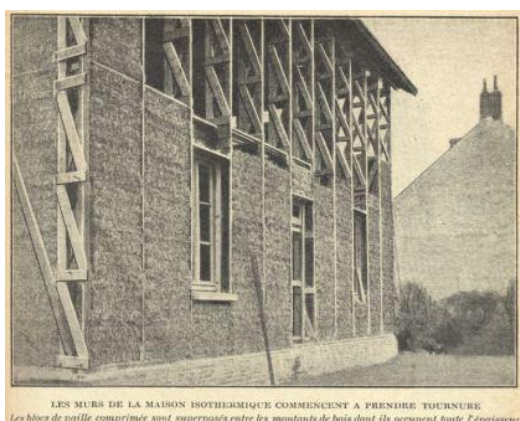
Fig 18 The historic Feuillet House in Montargis near Paris, built in 1920, uses simple truss frames between bales.
