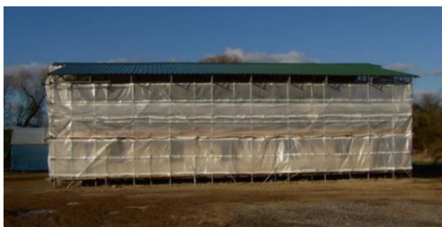
Fig 26 Example of rain and weather protection on site for bale storage and construction. This arrangement also provides protection for the lime during application and carbonation 47
