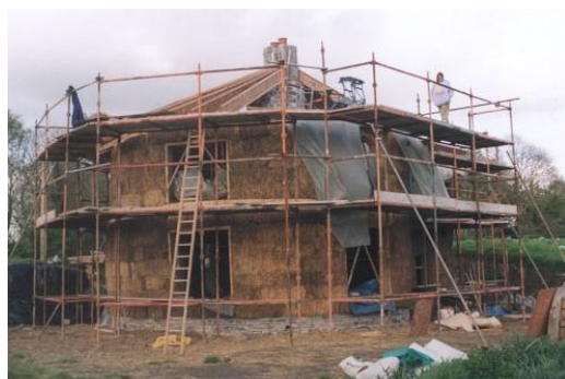
Fig 17 An example of 2 storey loadbearing construction showing cement-free foundations (limestone laid with lime mortar) with a timber ringbeam at ground, first floor and eaves level. Photo by Barbara Jones of the Spiral House, County Mayo, Ireland 2001.
