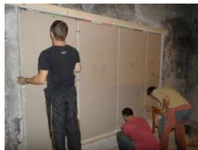
Clay plaster, straw wall with panels
